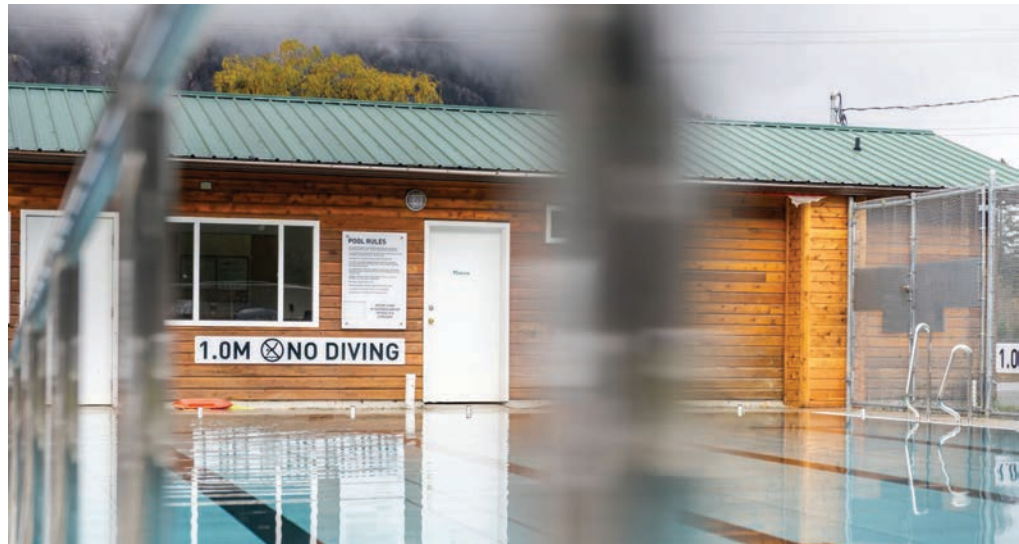
Durable stainless steel and easy maintenance let the community manage unpredictable spring openings, without the challenges that delay typical outdoor pool operations.
