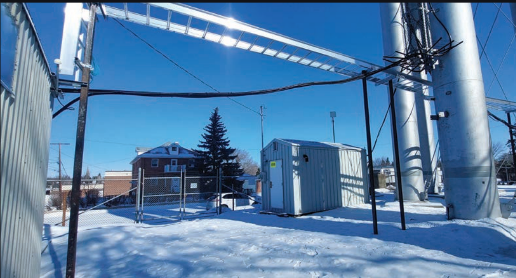
Instead of burying the cables, the project team is using a cable tray system to safely house and protect the wiring above ground.
