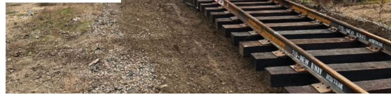
Above: The project involved cutting and removing the old track, followed by excavating the existing ballast to a depth of eight inches. Photos courtesy of Ralph Sjodin.
