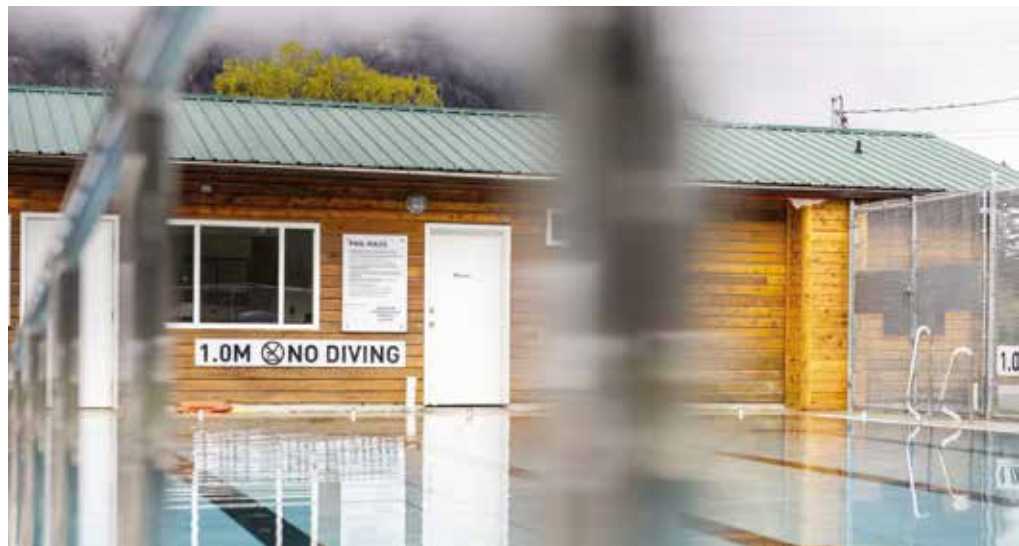
Durable stainless steel and easy maintenance let the community manage unpredictable spring openings, without the challenges that delay typical outdoor pool operations.
