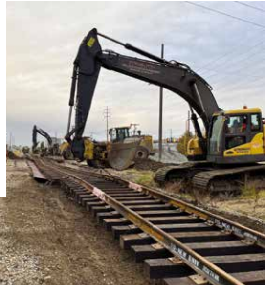
Above: The project involved cutting and removing the old track, followed by excavating the existing ballast to a depth of eight inches. Photos courtesy of Ralph Sjodin.
