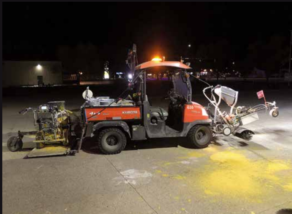
Public Works in Winkler, Manitoba, has used in-house ingenuity to convert a Kubota RTV900, making paint road markings safer and more efficient than it used to. Photo courtesy of City of Winkler.
