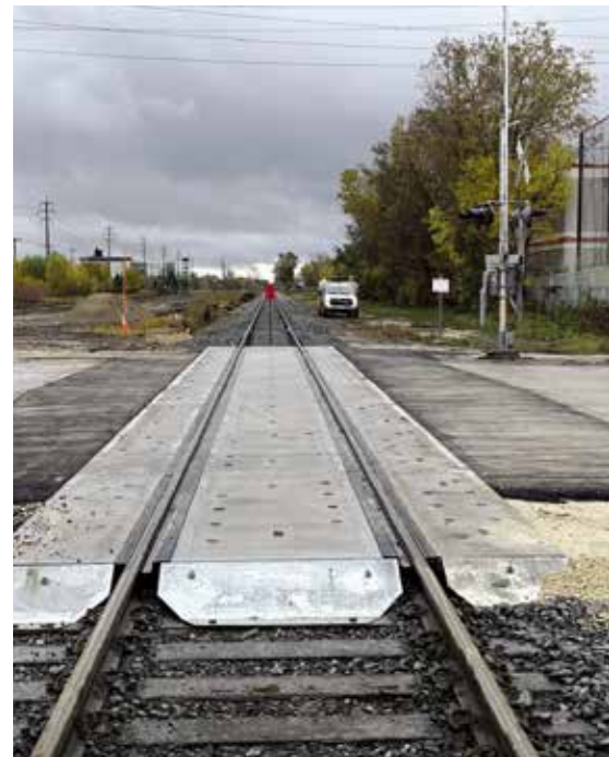
Below: The work done has improved safety and performance for rail freight, motorists, cyclists, and pedestrians for many years to come.
