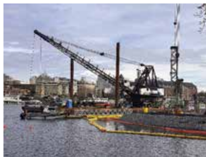
A floating crane working in Victoria's harbour. Photo courtesy of Peter McDowell.
