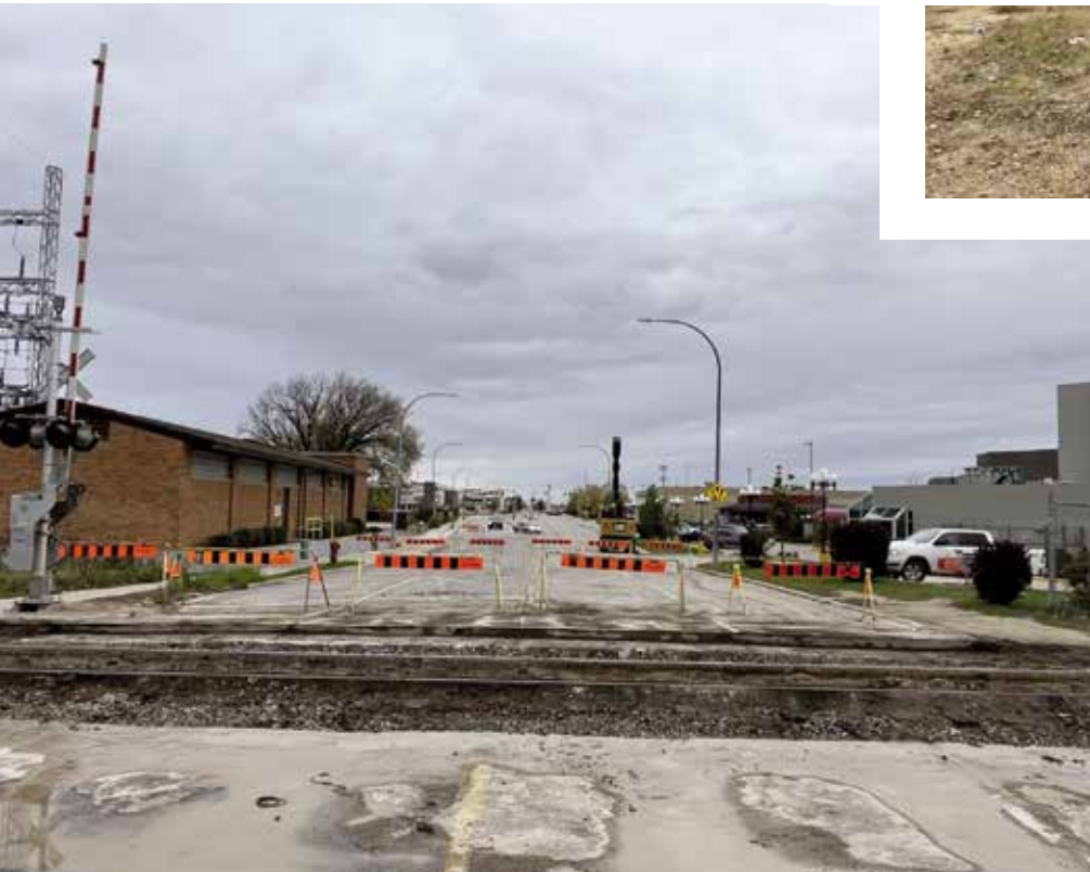
Above: The project involved cutting and removing the old track, followed by excavating the existing ballast to a depth of eight inches. Photos courtesy of Ralph Sjodin.
